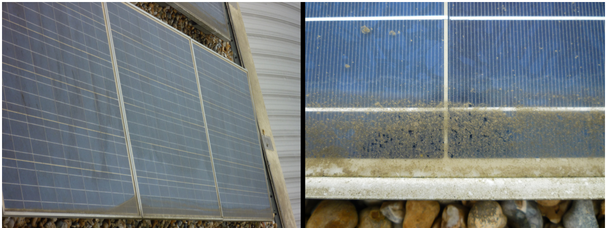
Figure 19: Dirt build up on lower edge of three PV panels (left) and close-up on one PV panel (right) situated on the SL roof.
